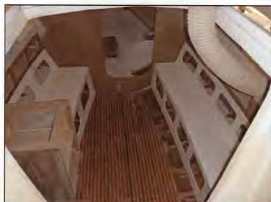
The new cabin interior.
