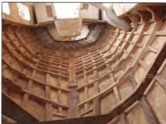
Interior looking forward showing the replaced ribs
