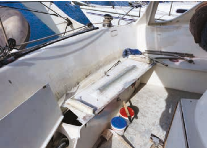
Sanding and priming of external surfaces
