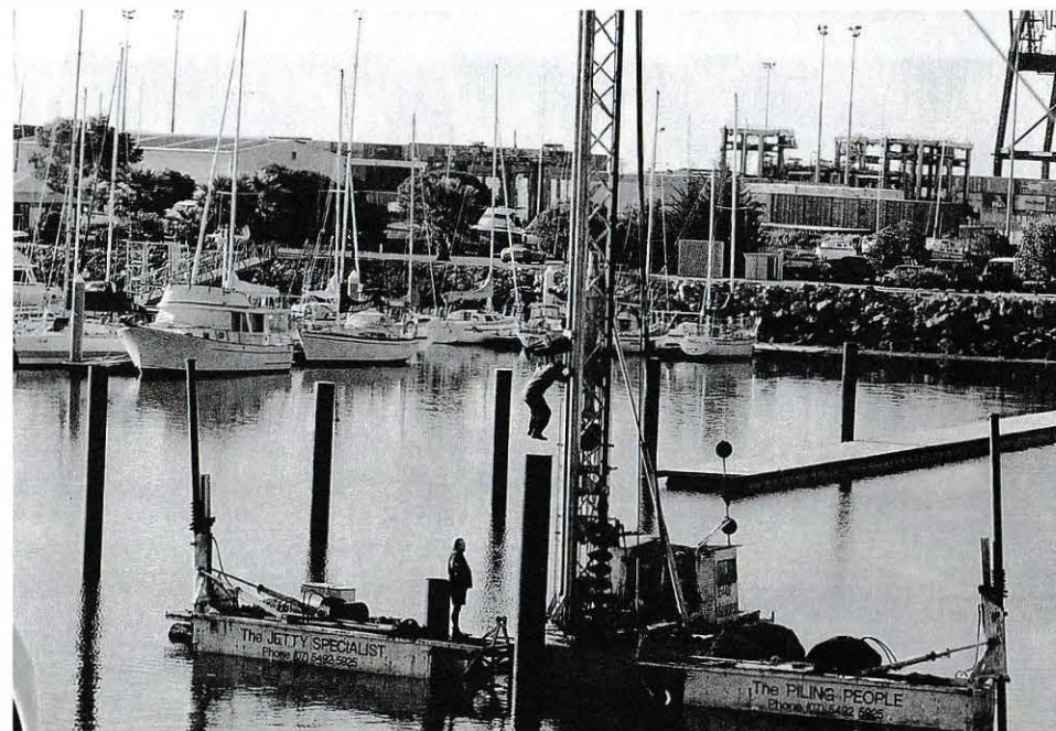
Remarkable agility and strength were required to place piles for the marina development. Peter and Helen White managed to capture a worker in midair. When the job was repeated, a conventional pile driver was used.
