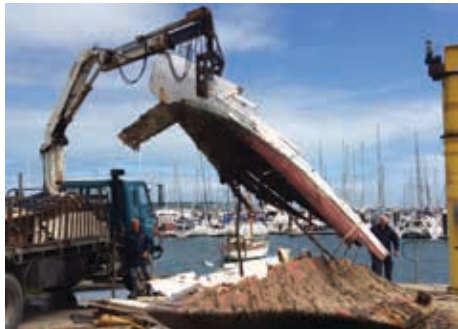
Being broken up - Sep 2016
