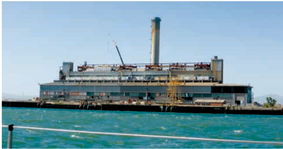
Playford/Alinta Power Station
